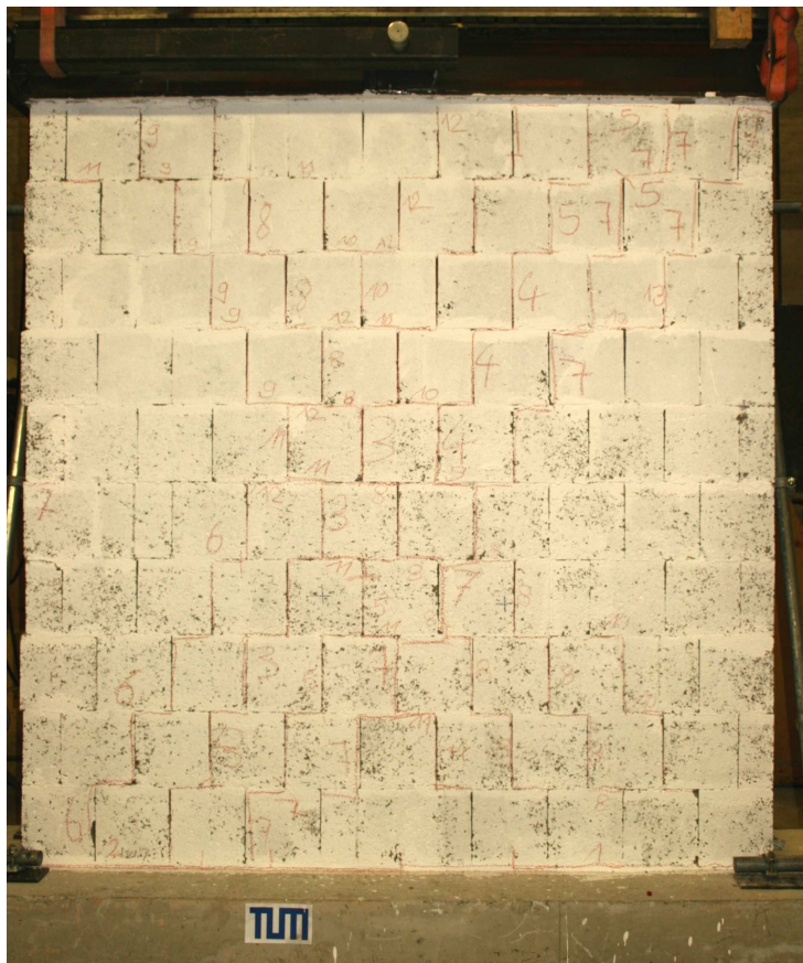
Figure 173: Crack pattern LAC03
