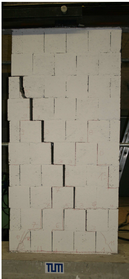
Figure 144: Crack pattern LAC01
