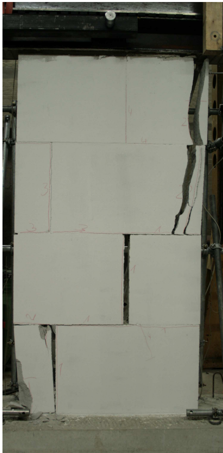
Figure 100: Crack pattern CS14
