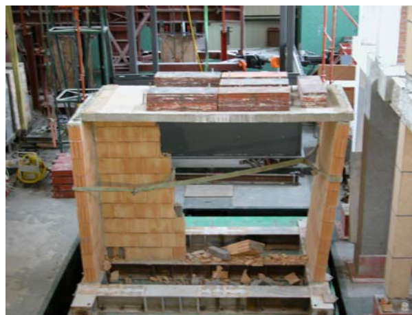
Figure 33. Specimen B2** : Damage at the end of tests.
