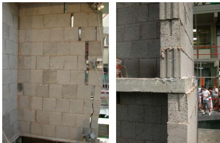
Figure 39. Specimen B4: Test 0.22g: Cracking through the height of 1 st level horizontal wall, crushing of lightweight concrete blocks and separation between transversal and horizontal wall of T- shaped part.
