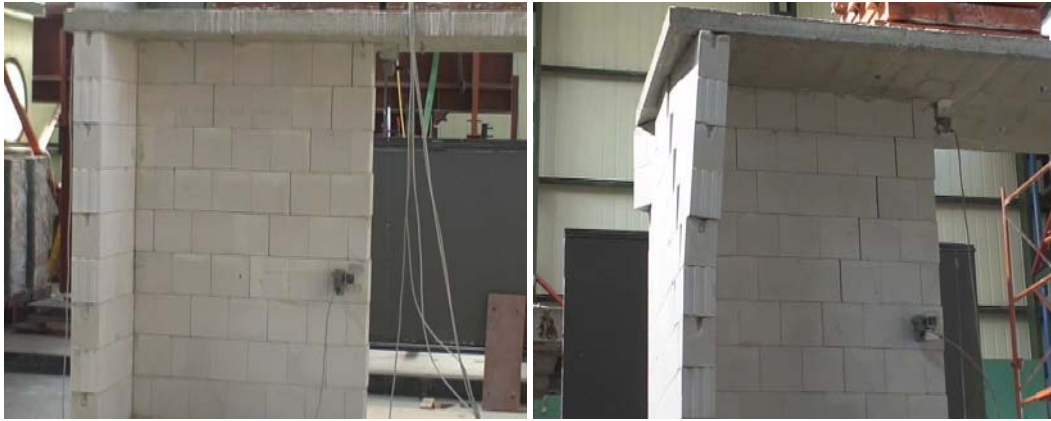
Figure 24. Specimen A1: Diagonal cracks of 1 st and 2 nd level - in plane walls.
