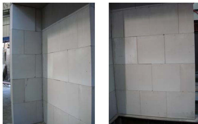
Figure 30. Specimen A3- with masses: Crack at the interface between transversal and horizontal wall of T- shaped part, crushing of units, diagonal cracks on horizontal wall.
