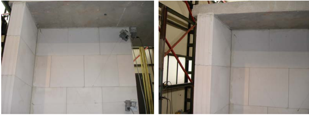
Figure 26. Specimen A2: Horizontal and vertical cracks of 2 nd level in plane wall.
