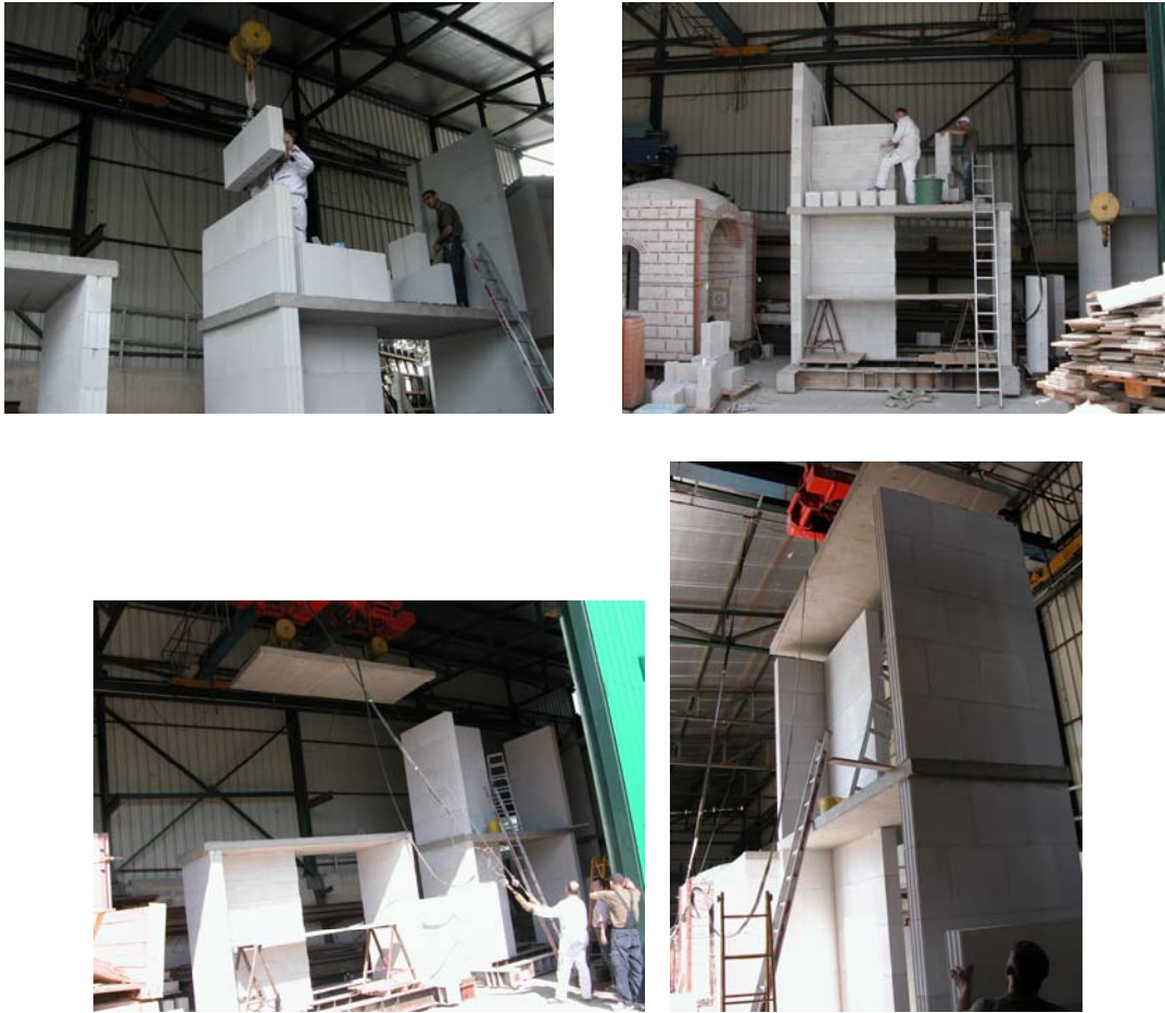
Figure 5. Construction of calcium silicate masonry buildings.
